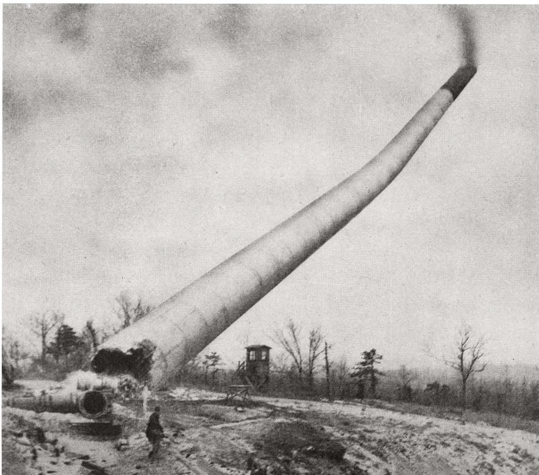
**IN ONE PIECE**—This big stack at Parlin, N. J., lasted but five years. It served a powder plant in wartime, and was razed to make room for a new plastics factory. That's not a last defiant puff; it's only dislodged soot.
